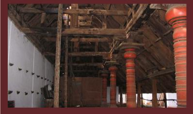
THIS PAGE Velyambalam; Extensive woodwork and reinforcement of wooden members has been used in the conservation
